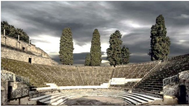
Fig. 8. View of the Roman theatre of Pompei highlighting the presence of the ambulatory and the gallery on the western side of the cavea .
