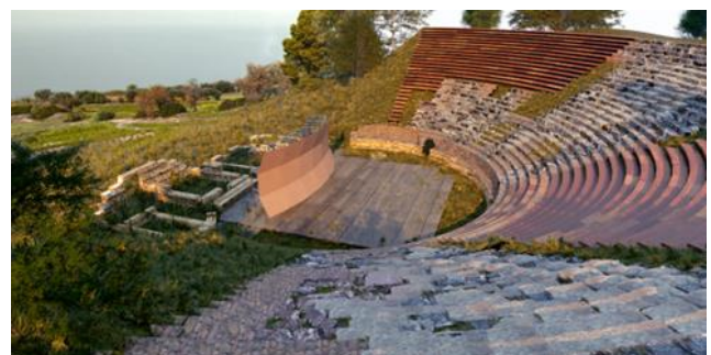
Figure 3 – Rendering of the 3D model of the theatre in the current state with the addition of an acoustic shell.
